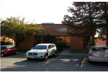
Mississauga condo unit Ideal for warehouse, mfg. uses
