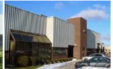
9,232 SF, 200 amps, 1 TL door 11% office, quick 410 access
