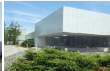
331,164 SF, 100 trailer spaces 4000 amps, 24 TL, 4 rail doors
