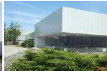
331,164 SF, 100 trailer spaces 4000 amps, 24 TL, 4 rail doors
