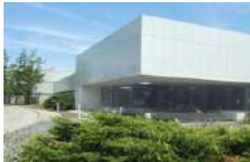
331,164 SF, 100 trailer spaces 4000 amps, 24 TL, 4 rail doors
