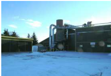
14,000 SF for wood industries 1,600 amps, equipment avail.
