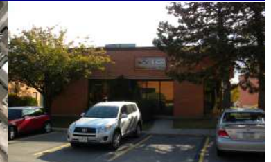
4,737 SF freestanding condo 2 truck level doors, 200A/600V
